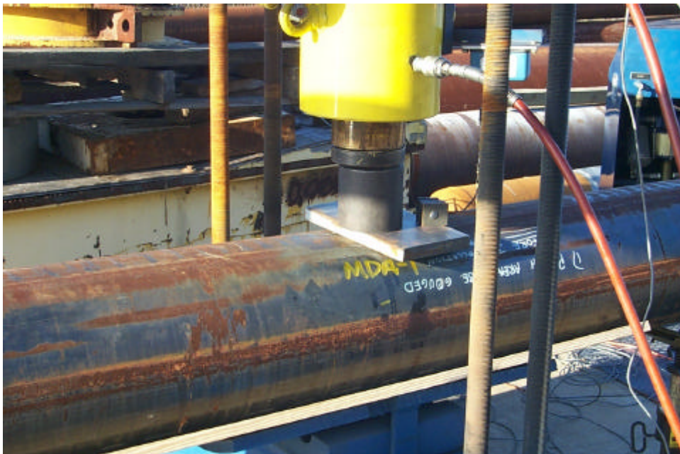
Figure 2 Close-up view of indenter plate creating dent in pipe
