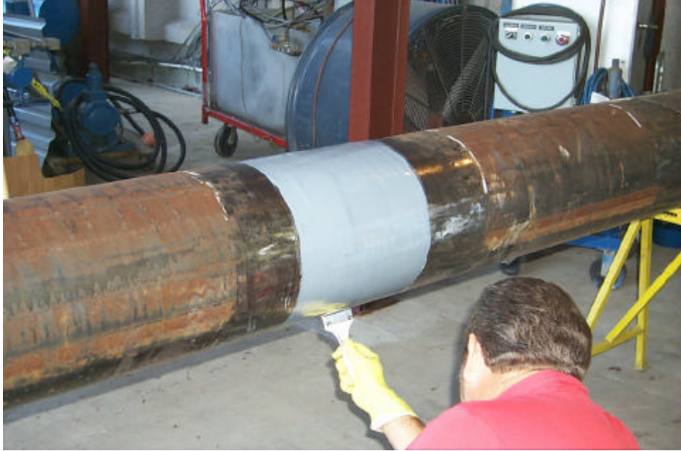
Figure 5 Application of epoxy primer
